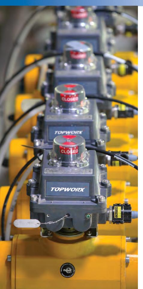
TopWorx<sup>™</sup> discrete valve controllers enable automated on/off valves to communicate via FOUNDATION Fieldbus, DeviceNet, AS-Interface, Profibus, HART and Wireless HART protocols. They attach to all rotary and linear valves and actuators, operate in the most demanding environmental conditions, and carry a variety of hazardous area certifications.
